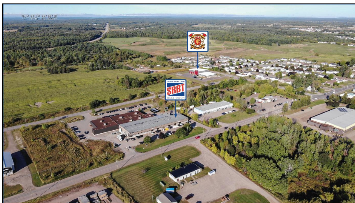
Figure 3: West view from the SRBT facility with Pembroke Fire Department shown.
